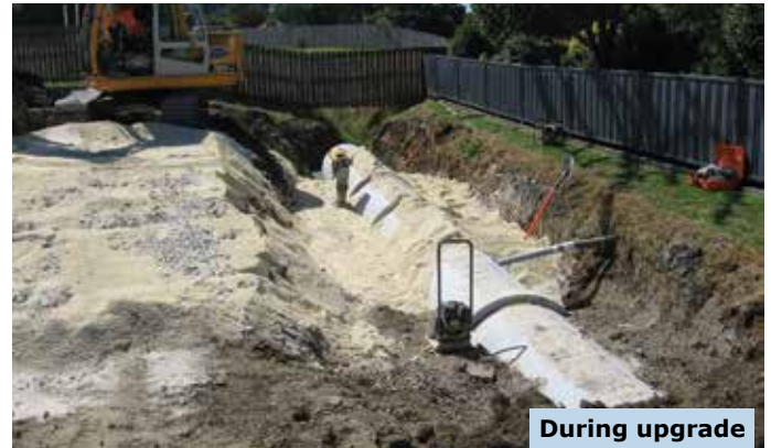
The upgrade of the St Andrew's Court Te Kuiti stormwater drain provides extra drainage needed to mitigate surface flooding at times of heavy rainfall.
