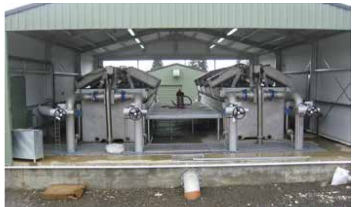
The upgrade of the Te Kuiti Wastewater Treatment Plant includes the implementation of treatment processes to enhance the overall function of the Plant; such as the sand filter (above) and a biological sludge reactor (below).
