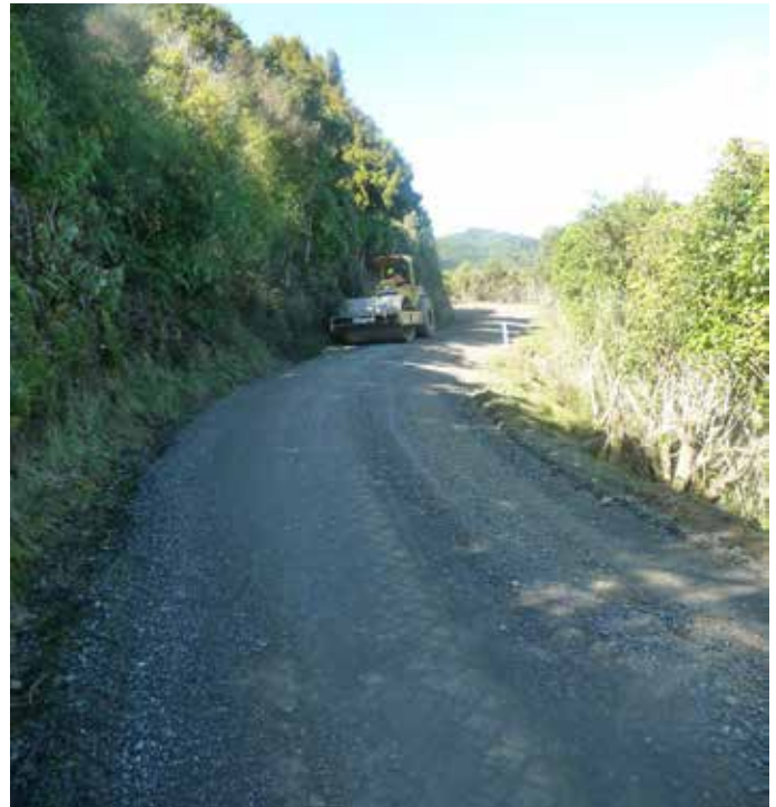
WDC's roading contractor Downers, carry out pavement rehabilitation works on a rural road in the Waitomo District.
