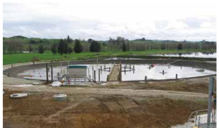
The upgrade of the Te Kuiti Wastewater Treatment Plant includes the implementation of treatment processes to enhance the overall function of the Plant; such as the sand filter (above) and a biological sludge reactor (below).
